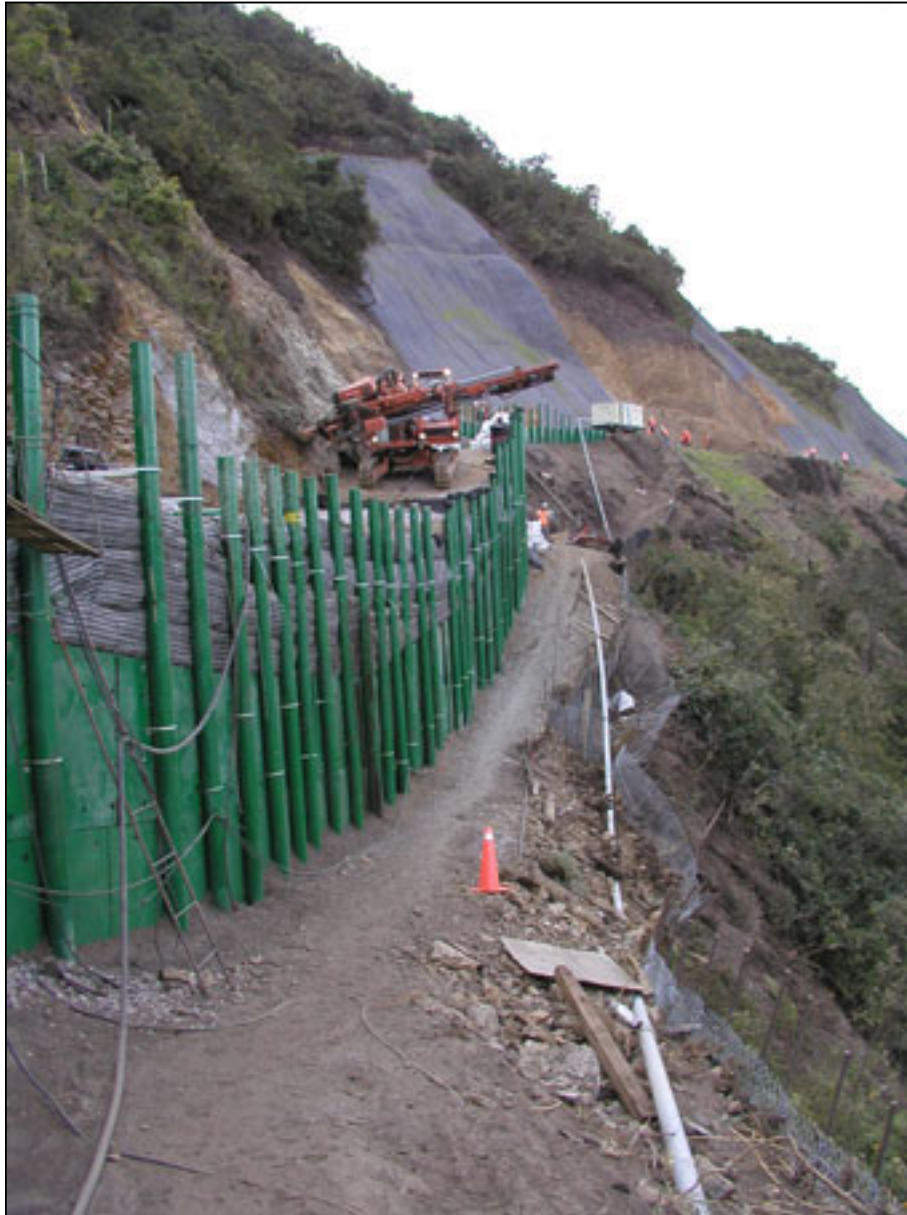
Image 10: Access road to Chiquilpe Pressure Reduction Station. The construction work already caused landslides on the steep mountain slopes (in the background covered with plastic sheet). The area is the habitat of the worldwide critically endangered Black-breasted Puffleg hummingbird (population est. 250 individuals).
